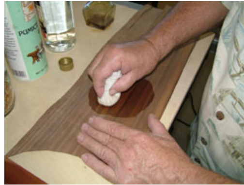
A thin coat of shellac is applied to the instrument, here represented by a piece of veneer.
